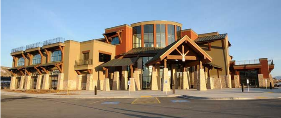
THE NEW CENTER OF EXCELLENCE (photo courtesy of USSA)
